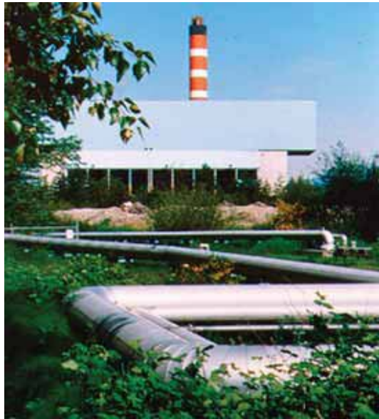
Figure A.1 Metro Vancouver WTEF facility with line that carries steam to adjacent paper recycling facility
